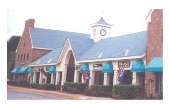
A retail store that uses a cupola as a focal point. Changes in the rooflines help to break up the mass of the building.
