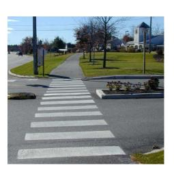
An island provides a refuge zone for pedestrians crossing this wide driveway. Flush unit pavers or textured asphalt crosswalks could have minimized annual maintenance
