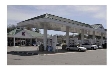
Lighting should be considered as an integral part of the canopy design. The canopy fixtures are recessed so the light source is not visible and does not create 'hot spots' that are distracting to the passing motorist
