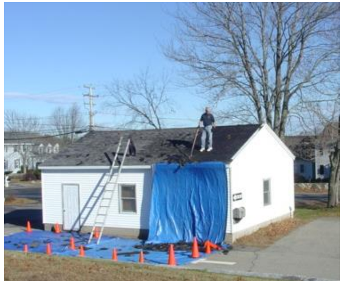
Chief Lord assists with removing old, weathered shingles for roof replacement to the Town Garage.
