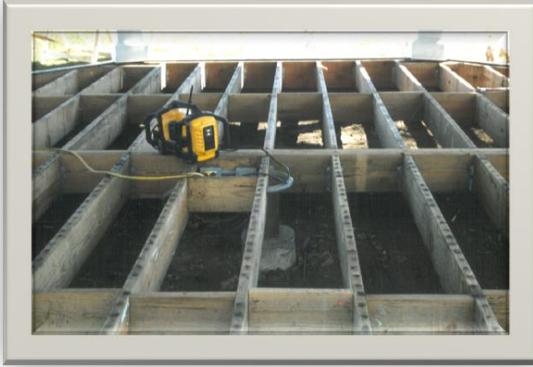
Decking removed from bandstand.
